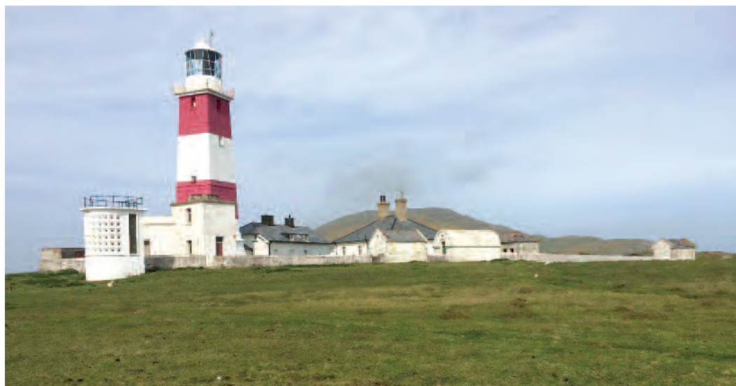
Figure 3. Bardsey Lighthouse and the perimeter wall that surrounds it, viewed from the south, May 2015. © Connor Stansfield.
